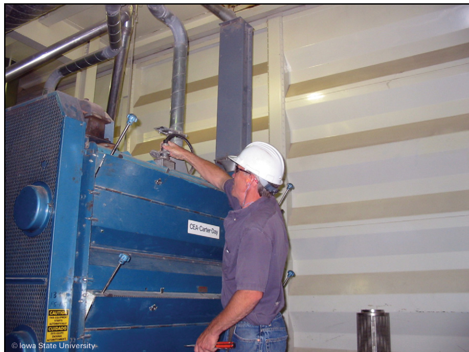
Figure 22. Disconnecting electrical power to rotary screen cleaner
