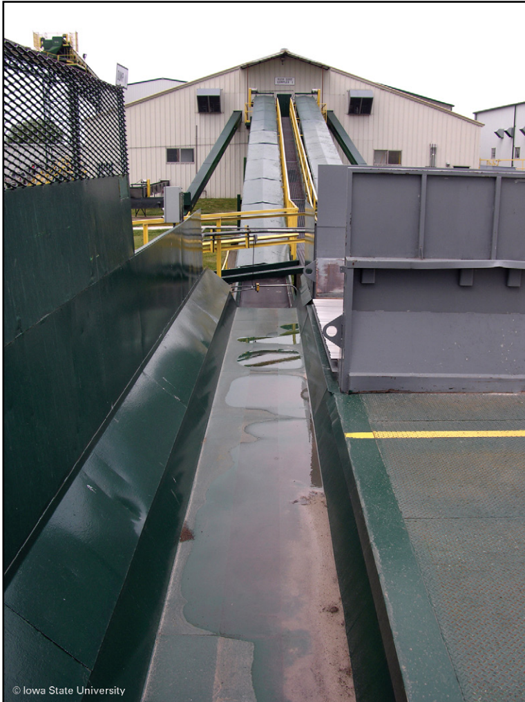
Figure 21. Receiving hopper for ear corn at a seed corn processing plant (truck unloads from empty bay on right into hopper and ears are moved on vibrating pan surface to flat conveyor belt in background)
