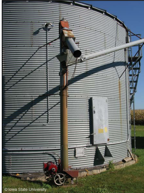
Figure 21. Unloading spout from conveying system on side of grain bin (note safety shielding is missing on lower auger drive)
