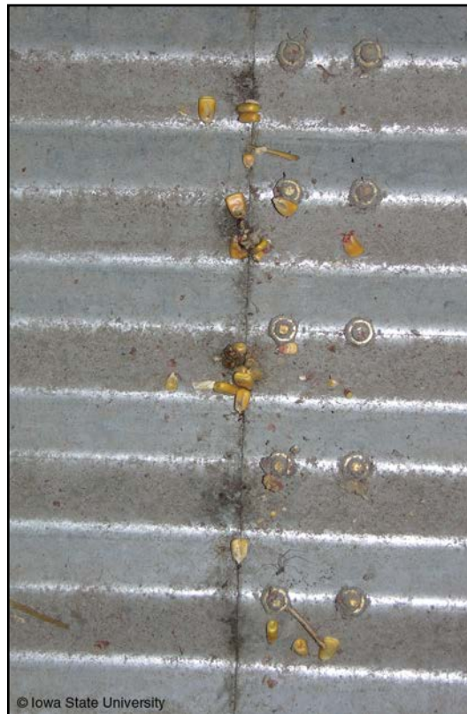
Figure 17. Grain adhering to interior bin wall surface
