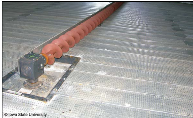
Figure 13. Mechanical sweep auger fastened to pivot around central sump (sweep auger is currently positioned over auxiliary sumps above unloading auger directly under bin floor)
