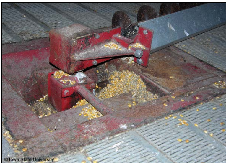
Figure 4. Sump for unloading in center of bin floor
