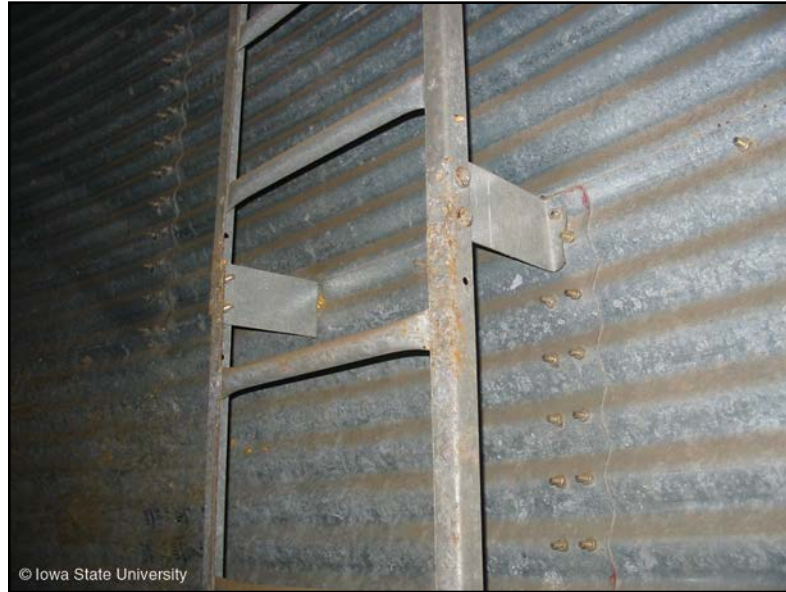
Figure 16. Support structure for interior bin ladder
