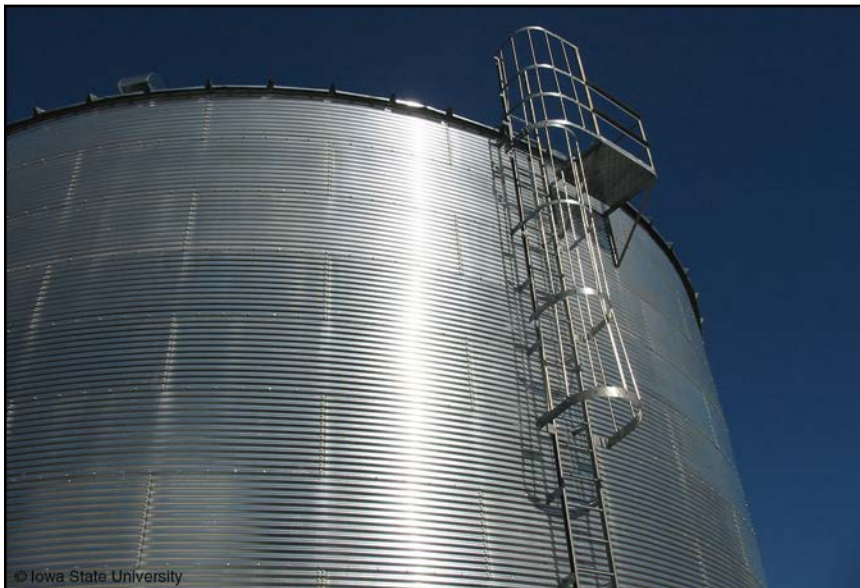
Figure 11. Ladder with safety guards to bin roof
