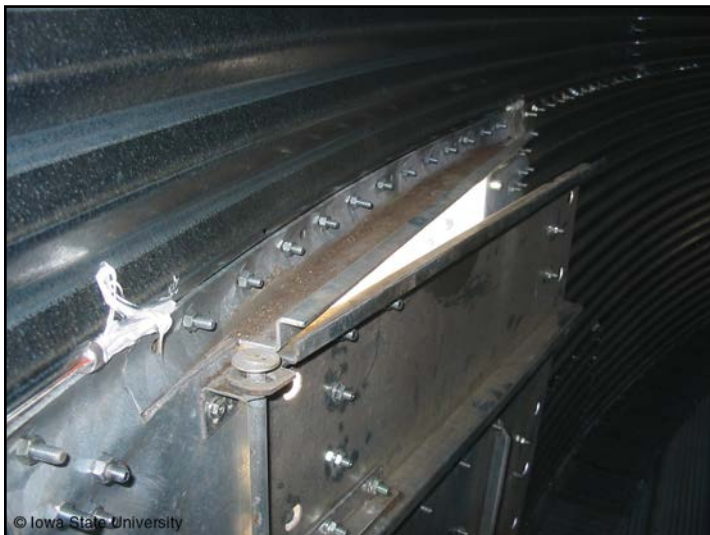
Figure 15. Interior horizontal flange above bin doorway
