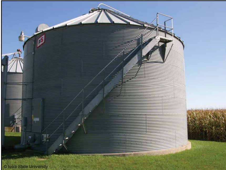
Figure 10. Access stairs to bin roof
