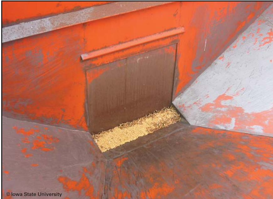
Figure 11. Retractable door for grain unloading (note two ledges above door opening)
