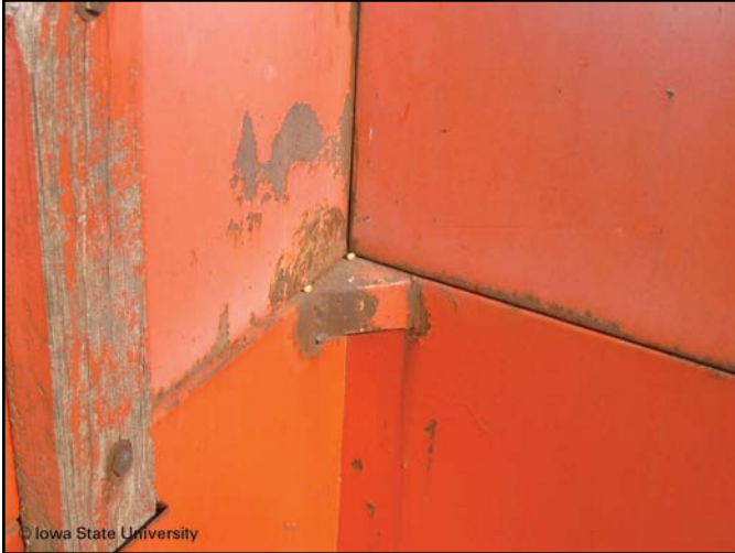
Figure 1. Structural flange at corner of grain box
