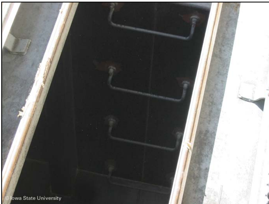
Figure 30. Interior access steps as viewed through top hatch
