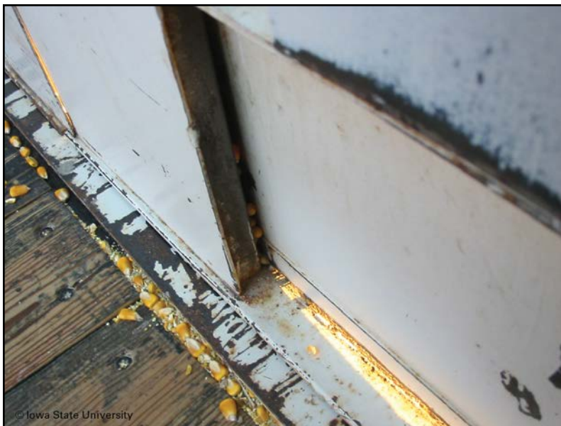
Figure 16. Residual grain near unloading door
