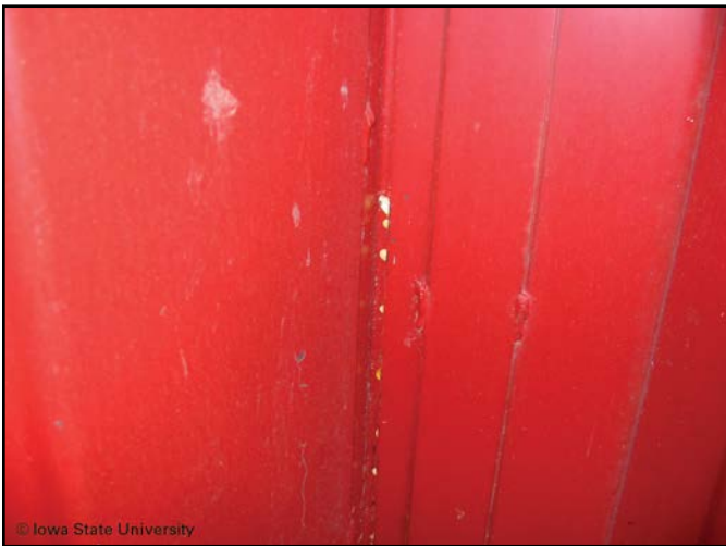
Figure 3. Seam of overlapped steel at corner of grain box
