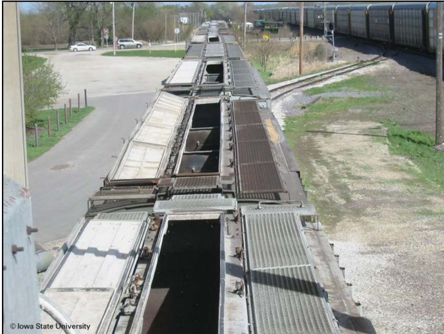
Figure 25. Open hatches on top of rail cars
