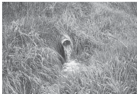
Concerns with present stream condition: Erosion and loss of cropland, tile drainage into the stream, and erosion by livestock.
