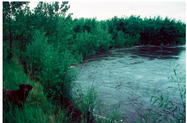
Three years later, the same area along Bear Creek has been stabilized by planting willow cuttings, trees, and shrubs.
