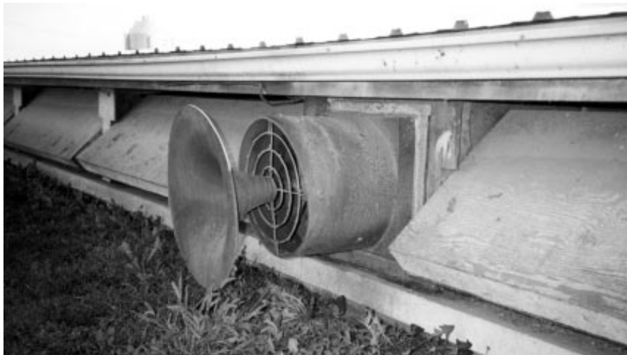
Photo C. A wind diverter is important for fans located on the north wall to reduce wind action on the fans, especially when they're run at slower speeds.
