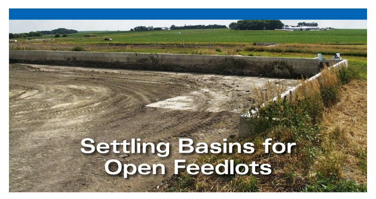
Separation of solids from open feedlot runoff is an important part of managing manure movement caused by rainwater and melting snow. Using gravity to remove solids by settling them to the bottom of a small pool (basin) is the most common and cost effective method for feedlot runoff solids separation.
