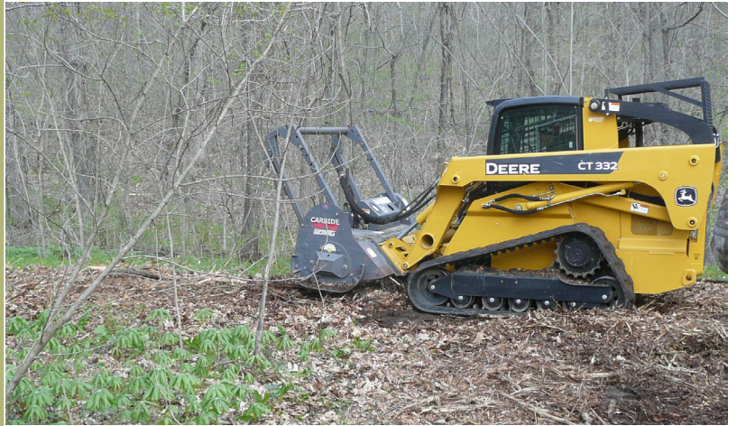
Forestry mower to create firebreak in existing woodlands
