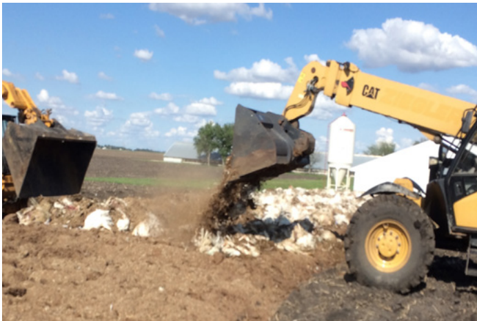
Figure 2. Combined materials being placed with a front-end loader and a telehandler from either side of the base without driving over it.
