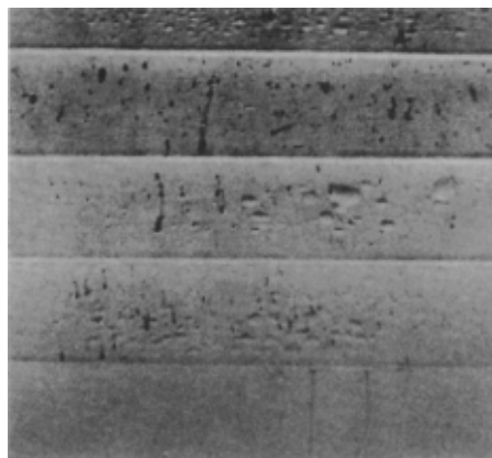
Figure 1. Moisture blistering and peeling.
