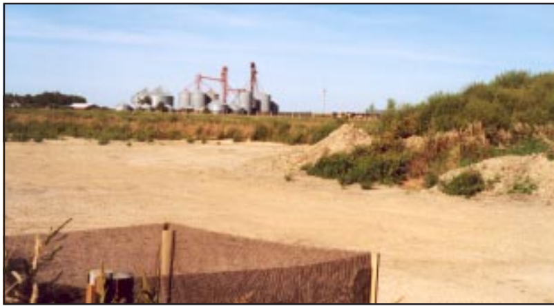
Manure solid settling basin at a feedlot in northwest Iowa.
