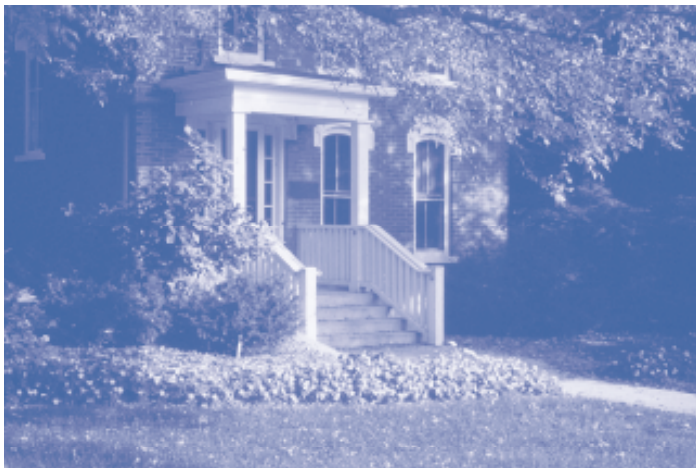
Figure 2. Front view of home entrance showing typical steps leading to front door
