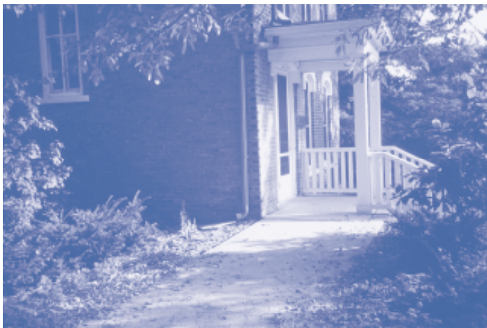
Figure 3. Side view of home entrance showing a no-step design integrated with surrounding landscape
